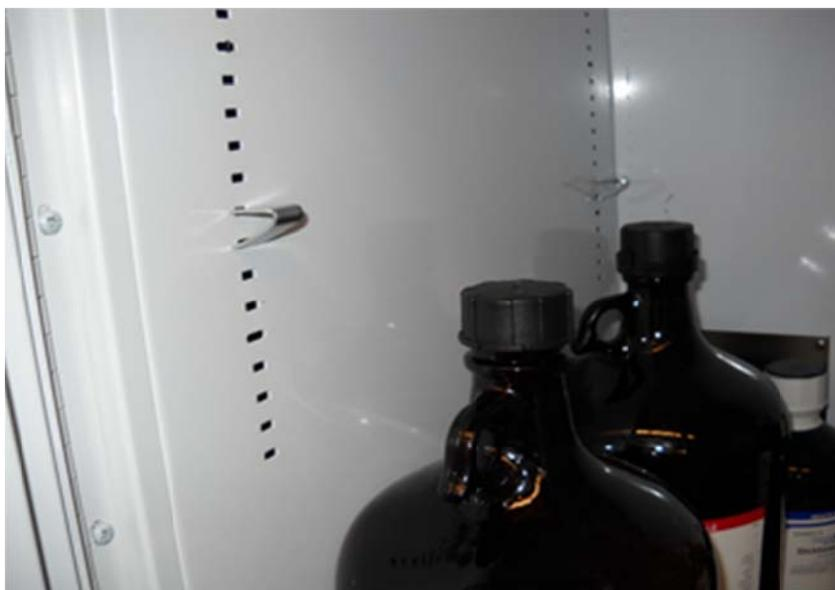
Another cause of shelving collapse is an overloaded shelf. Please remove chemicals from any storage shelf that appears to be bowing due to excessive load. An overloaded shelf will eventually drop because as it bows there is less shelving resting on the support brackets.
